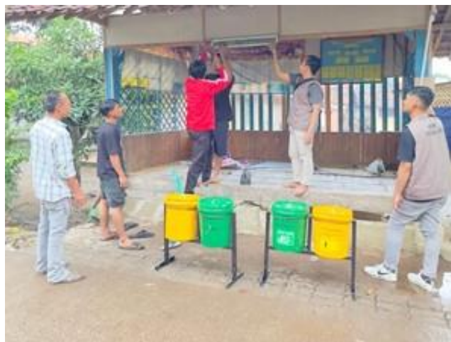
Gambar 3. Proses Pemasangan Text LED
